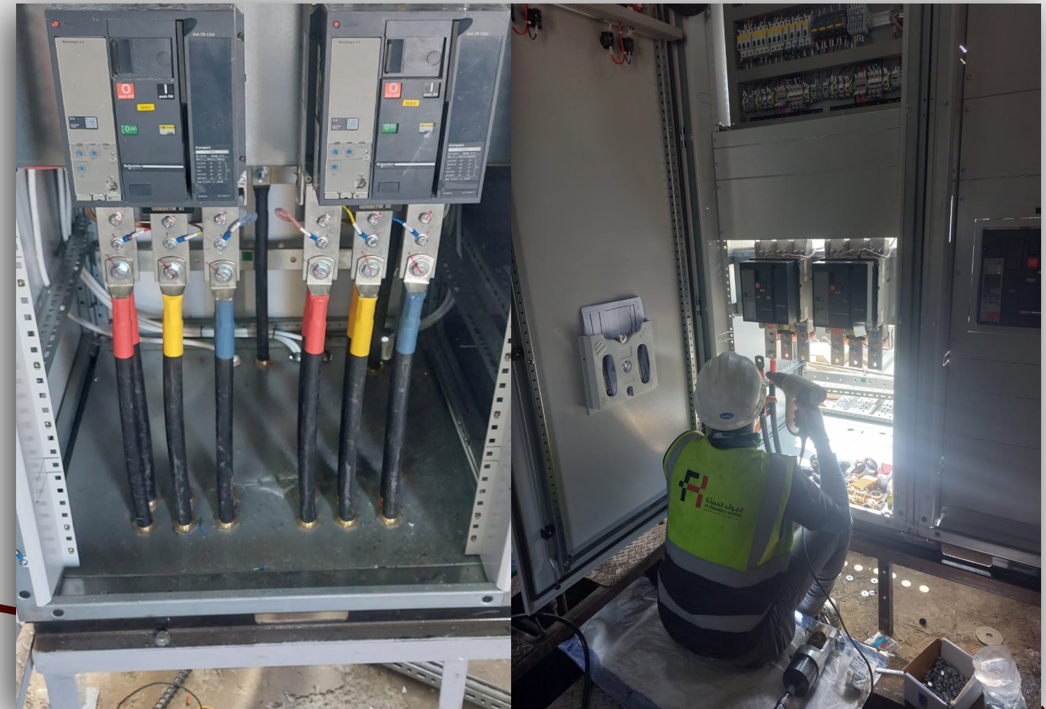
Generator Project for Azad Real Estate Company – Corniche Commercial Center
