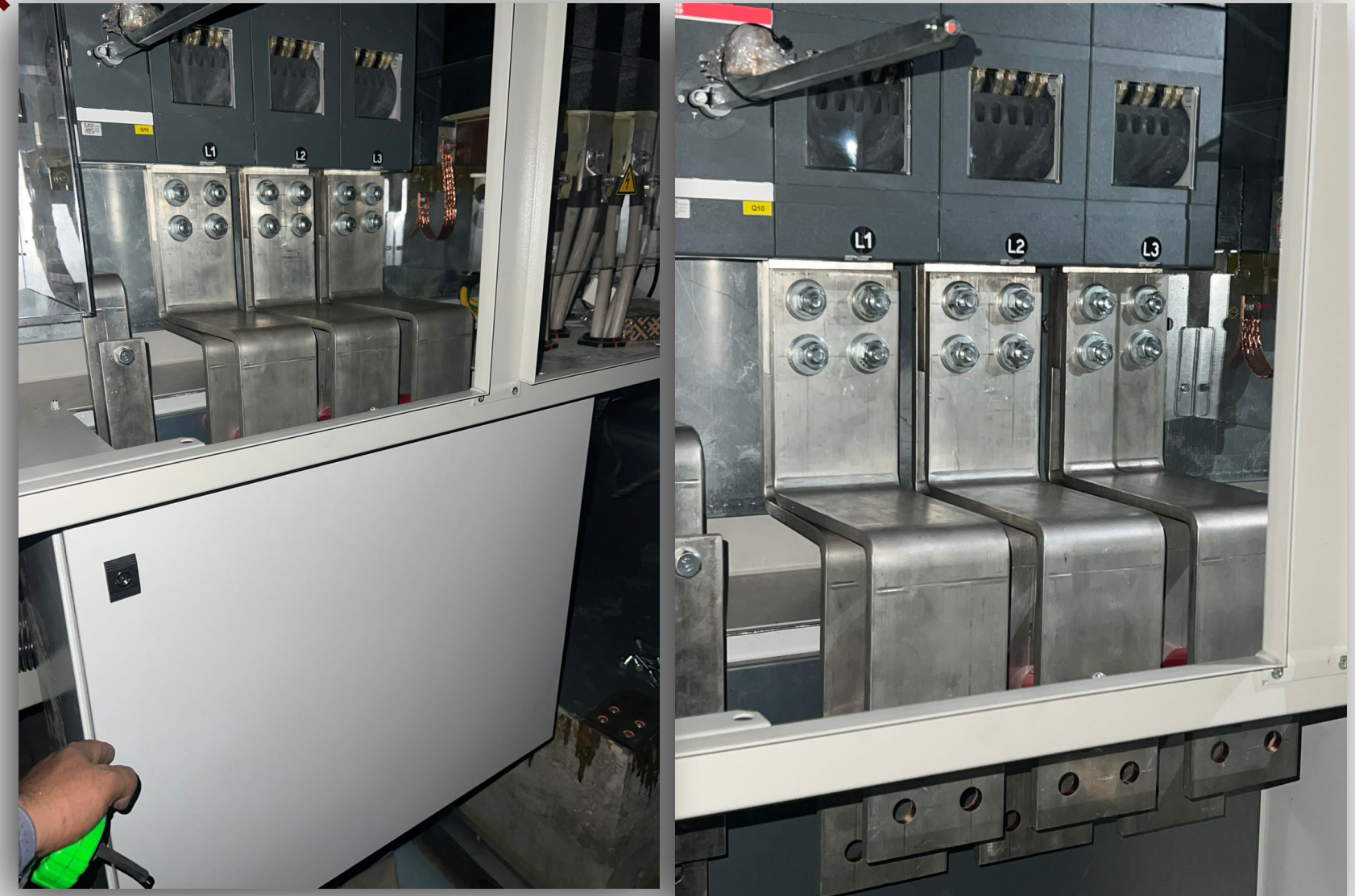
Fabrication and Installation of a Busbar Box – Al Huda Park, Makkah
