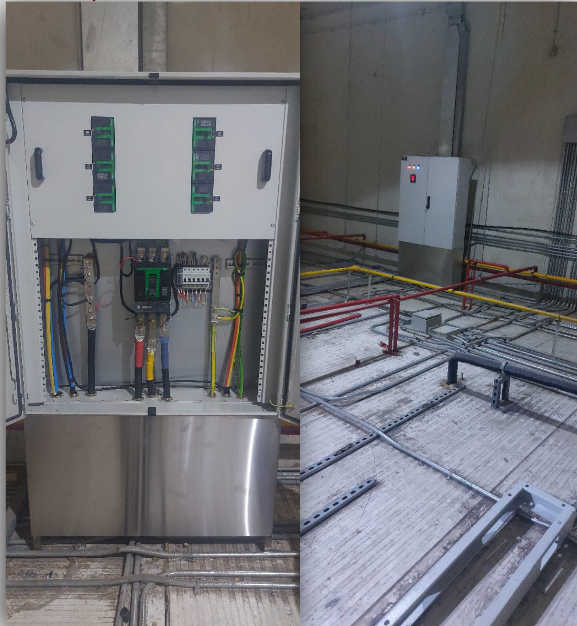
MDB Panel Installation with Cable Laying and Cable Tray Installation – Distinguished Foods Factory
